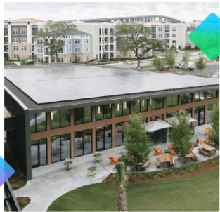
Solar panel farm at LEED Gold HQ in Charleston, SC
